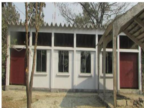
Figure 6. Pilot plant shed structure for Compressed Stabilized Earth Block (CSEB) production at HBRI campus
