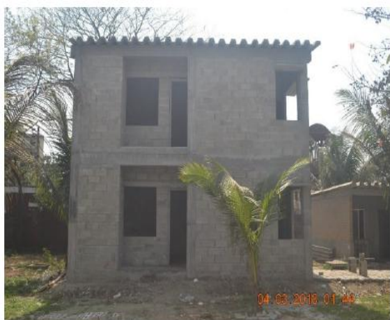
Figure 5. Model House-II using Compressed Stabilized Earth Block and Thermal Block at HBRI campus
