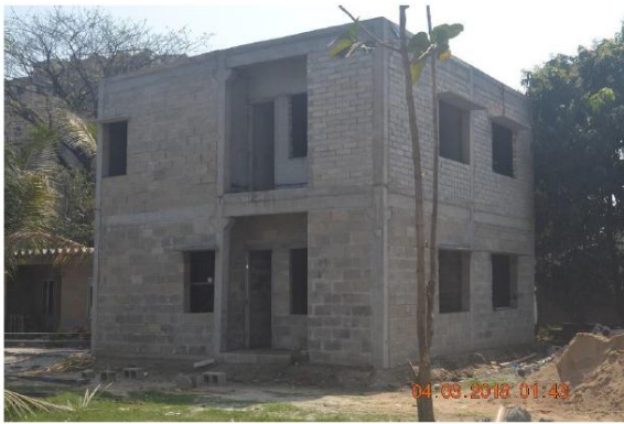
Figure 8. Model House-II using Compressed Stabilized Earth Block and Thermal Block at HBRI campus
